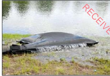
Plate 2-2 Silt Bag with water being pumped through
