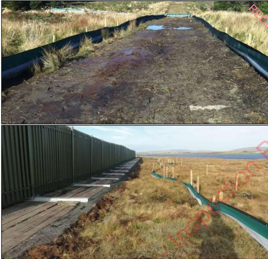
Plate 2-4 Typical Silt Fence Details
