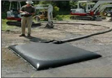
Plate 2-1 Silt Bag under inspection
